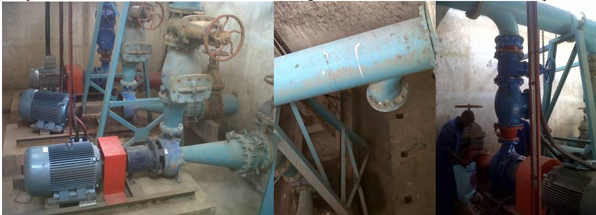
Pump Station 3 newly refurbished pump sets 1 & 2 and new installation 3 in the far end to the wall (photos 26). Photo 28 shows the new pump in greater detail.
