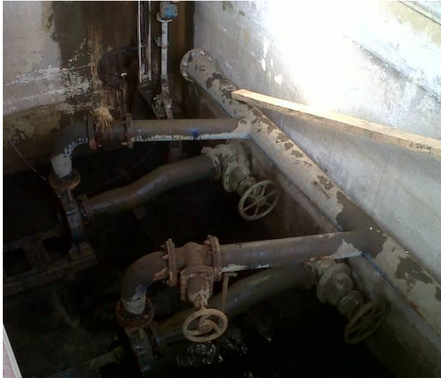
Pump Station No 1 showing once flooded equipment (left) photo 9 and operating new pumping gear in the drywell (photo 10)
