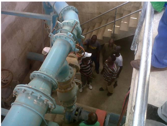
Pump Station 3 newly refurbished pump sets 1 & 2 and new installation 3 in the far end to the wall (photos 26). Photo 28 shows the new pump in greater detail.
