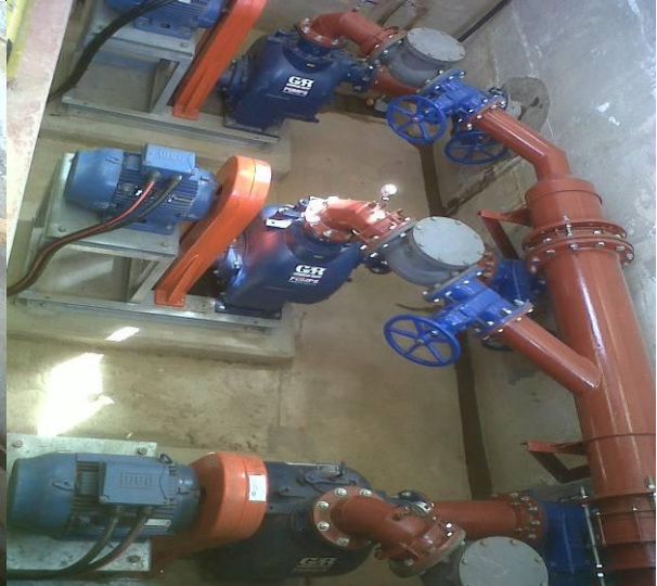
Pump Station No 1 showing once flooded equipment (left) photo 9 and operating new pumping gear in the drywell (photo 10)
