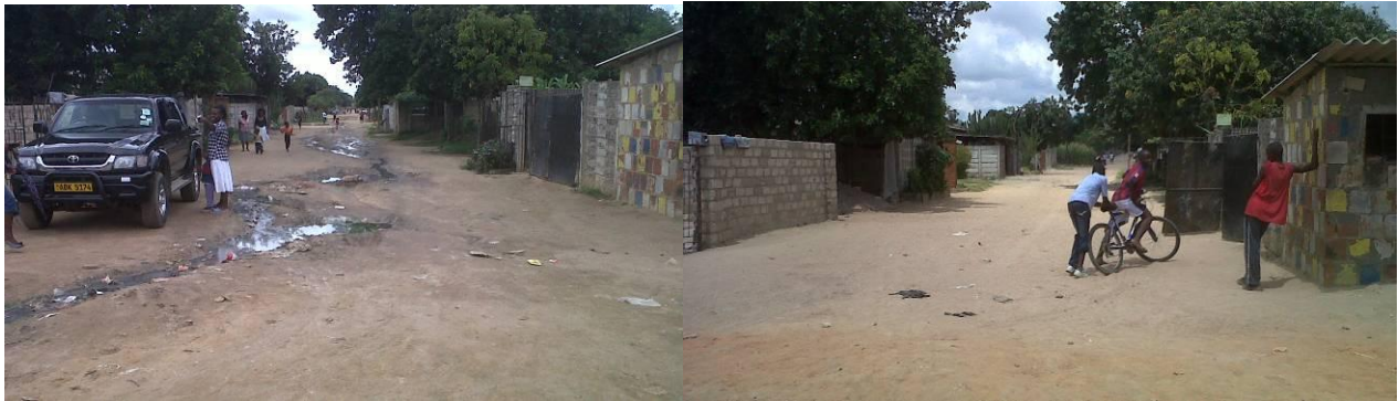
Photo 42: sewage overflow along Ruzvidzo Road before and after (photo 43) the intervention
