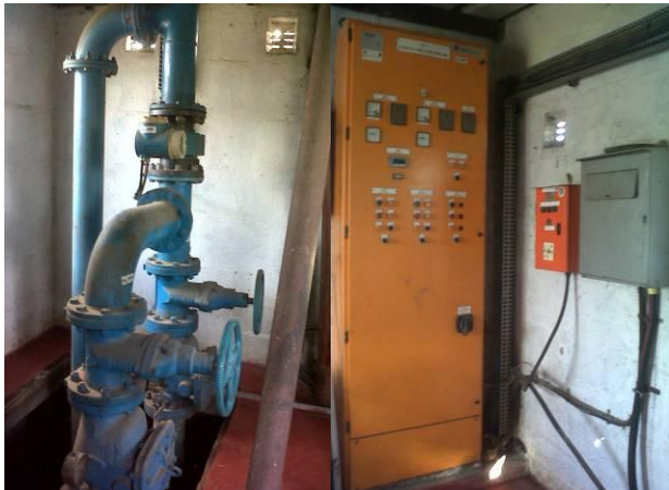
Pump Station No 2 showing existing piping and refurbished control equipment (left) (photo 11 & 12) and new submersible pumping gear (photo 13) and artisan fixing the new pump in the wet well (photo 14)
