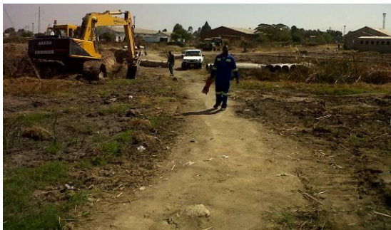
Photo 44: Sewer pipe replacement activity in progress
