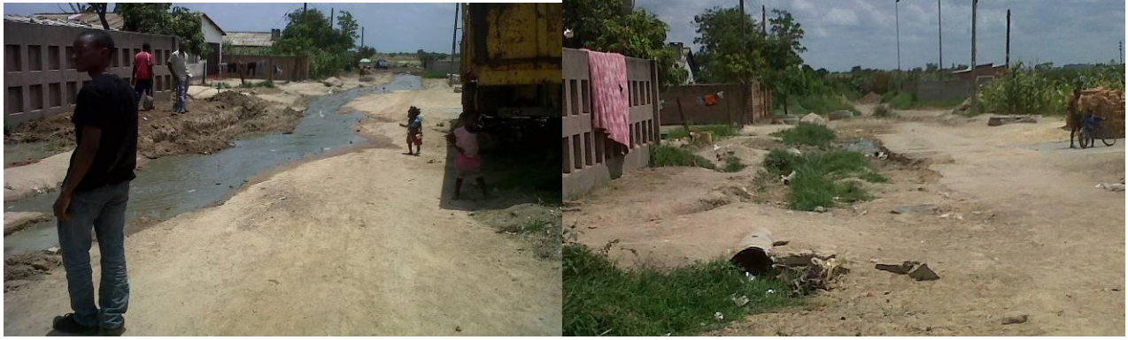
Photo 40: sewage overflow along Chiratidzo Road before and after (photo 41) the intervention
