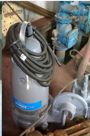
Pump Station No 2 showing existing piping and refurbished control equipment (left) (photo 11 & 12) and new submersible pumping gear (photo 13) and artisan fixing the new pump in the wet well (photo 14)
