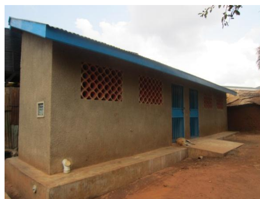
Picture 3-2: Public toilet in Kagugube
